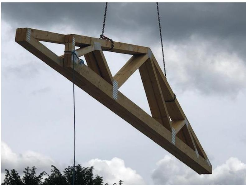
To integrate energy saving throughout the design, the flat roof was built over with a pitched roof. Photovoltaic panels were built onto the roof pitch as this provides a better angle of inclination for capturing the sun's light energy, converting to electricity. Natural sheep's wool insulation was laid inside the new roof space. Thermafleece was chosen as it is much less hazardous to lay, and also biodegradable.
